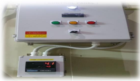
< Fig 4. Refrigeration warehouse >
