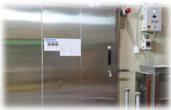
< Fig 3. Refrigeration warehouse >
