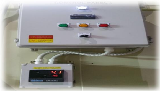
< Fig 4. Refrigeration warehouse >
