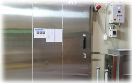
< Fig 3. Refrigeration warehouse >
